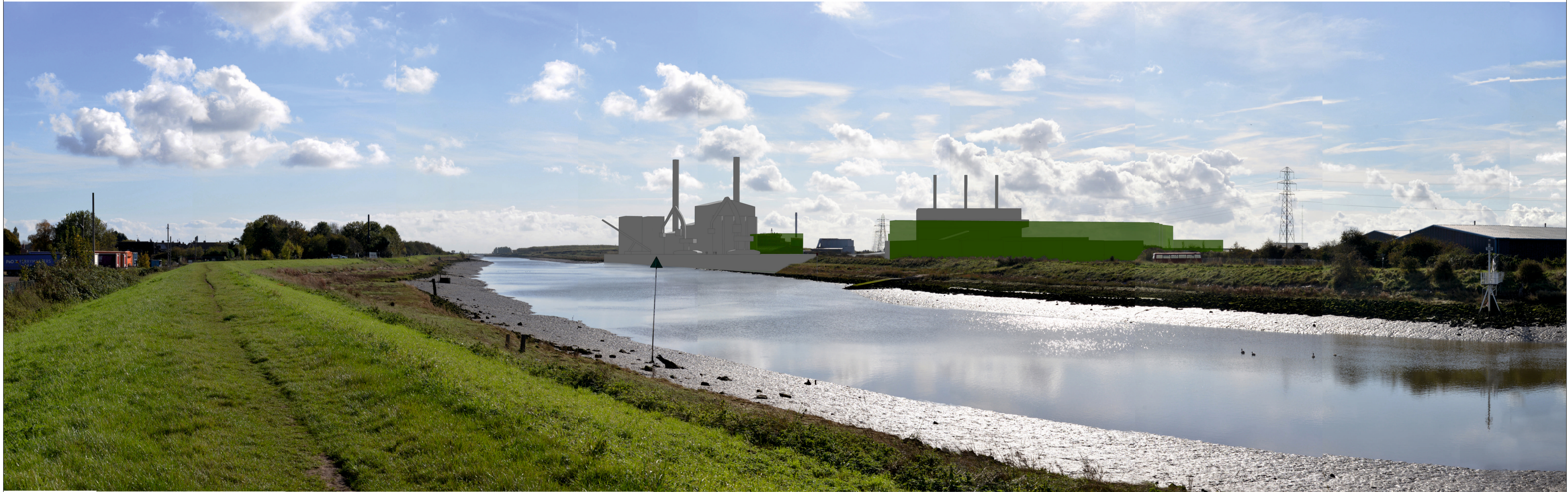
View 8: Photomontage view of the proposed Facility at Year 15 illustrating the potential effect of long term established woodland planting (green blocks)
